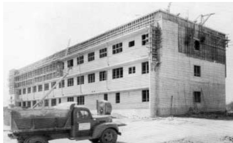
April 1951, construction is well underway.
