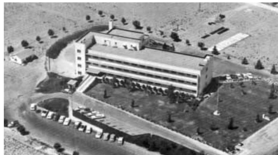
First phase of hospital construction is completed.
