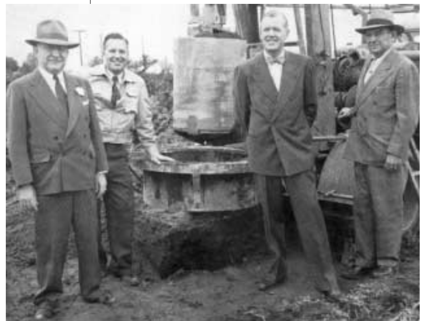
March 1948, taking earth-core samples for foundation tests.
